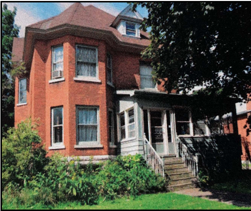
The first house to get water was the home of John Carruthers at 554 Henry Street West in Prescott.
