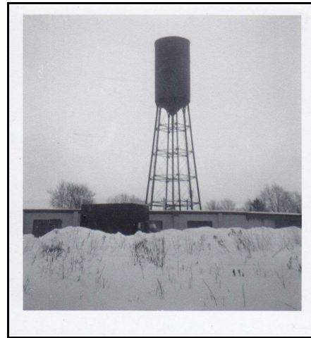
This water tower was the original built in 1889 and it was replaced in 1970 by a new cement one.
